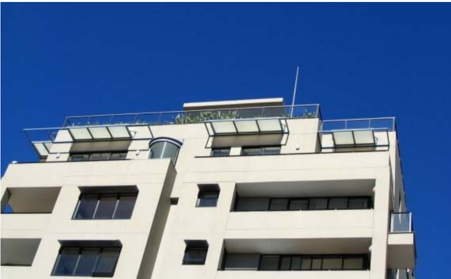
High rise building with glass infill safety railings
