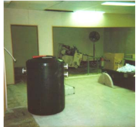
Fig 1. Canteen area. Concrete saw (background)
