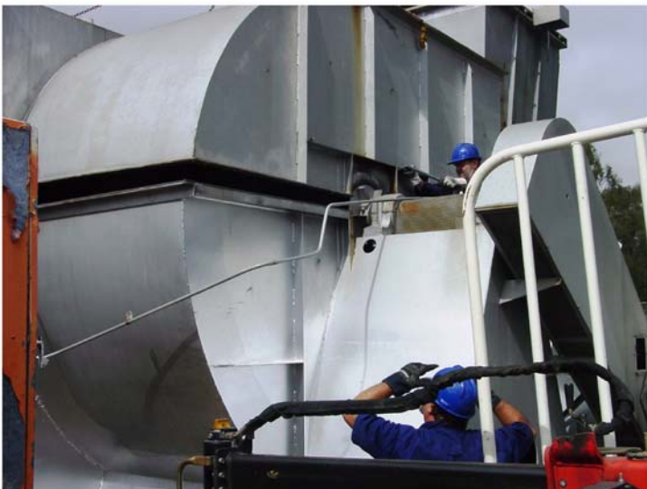
Paul, Dave & Stephen fitting the intermediate section of the fan assembly
