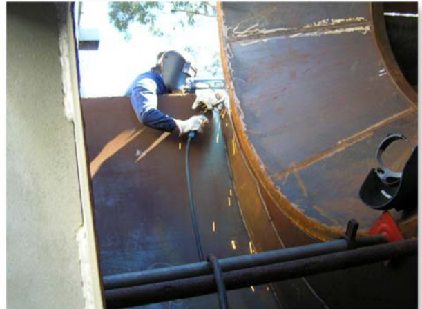
Paul welding in the replacement sections in the base
