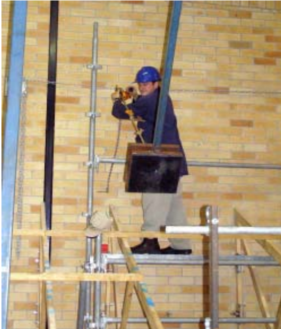
Joshua Kent preparing to test a new roof edge protection system
