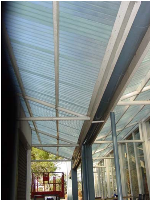
Building 17 rear awning roof replaced
