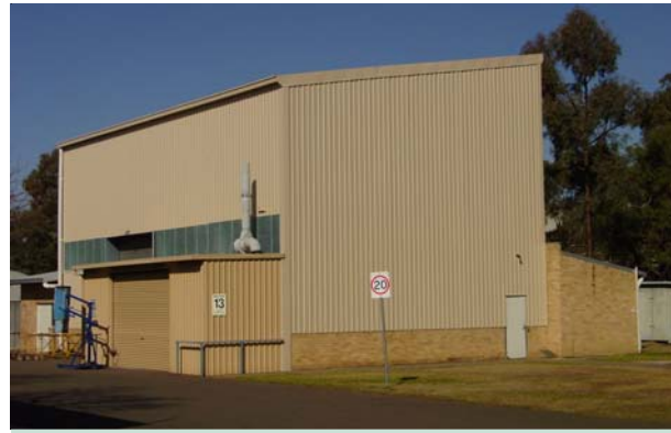
Building 13 completed with colourbond roofing and walls
