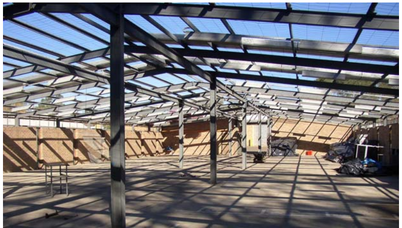
Building 10 after removal of asbestos roof cladding
