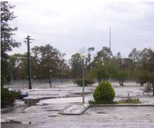
TestSafe drenched and damaged by the Spring Storm
