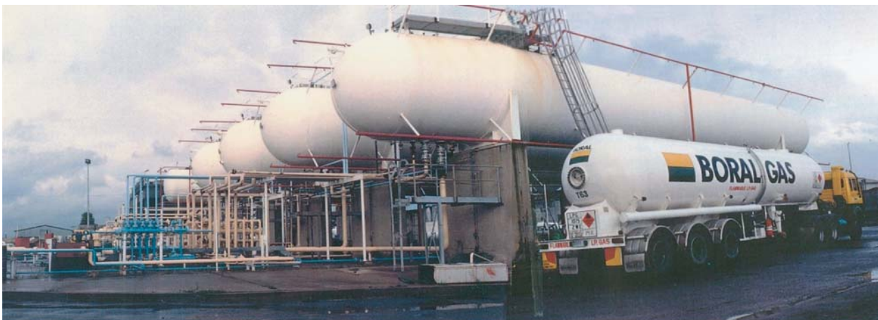
View of the LPG terminal before the explosion. Note: Red drencher pipes above and below each tank, and the LPG Road tanker in a similar position to that of the night of the explosion
