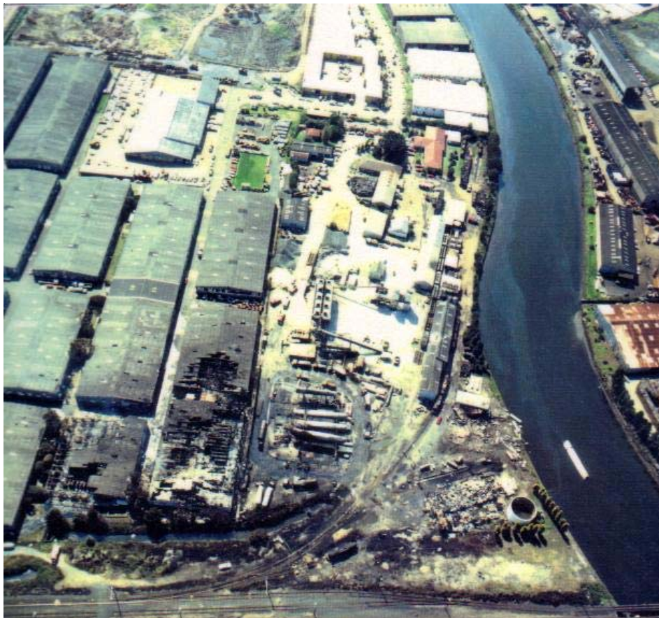
Arial view of the BORAL Gas site after the fire.
